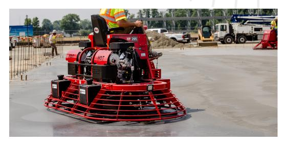
The HP205 is the most cost effective 10-footer in the industry. With the maximum amount of low-end torque, this machine is a great alternative to the more expensive T4 diesel 10-footers. The lower maintenance costs complement the affordablility of the HP205 rider, reducing the cost of ownership.
